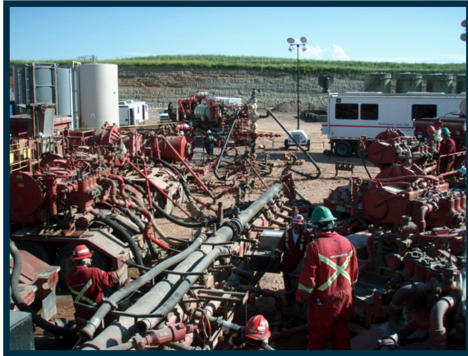
Figure 1-9: Fracturing trucks working together to inject well 5
