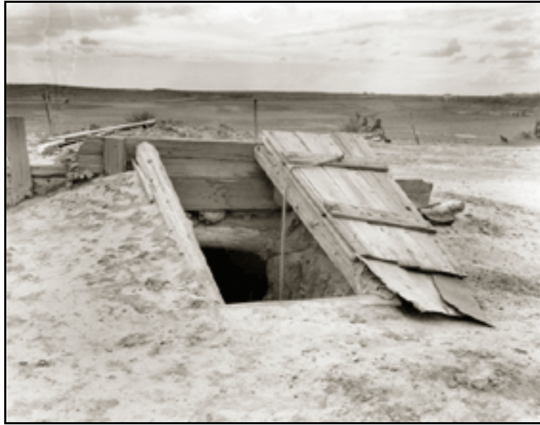
Storm cellar on the Texas plains, West Texas panhandle, June 1937
