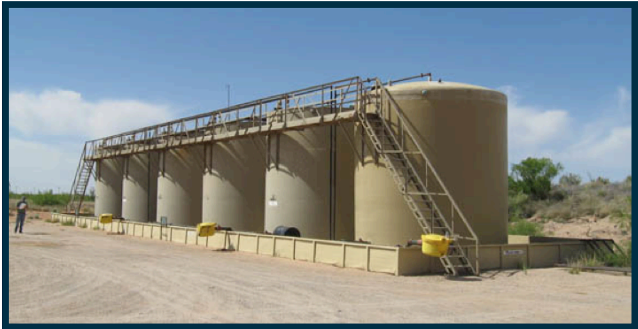
Figure 1-11: Tank battery 59
