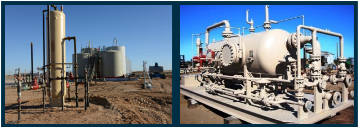
Figure 1-10: Oil separators 58
