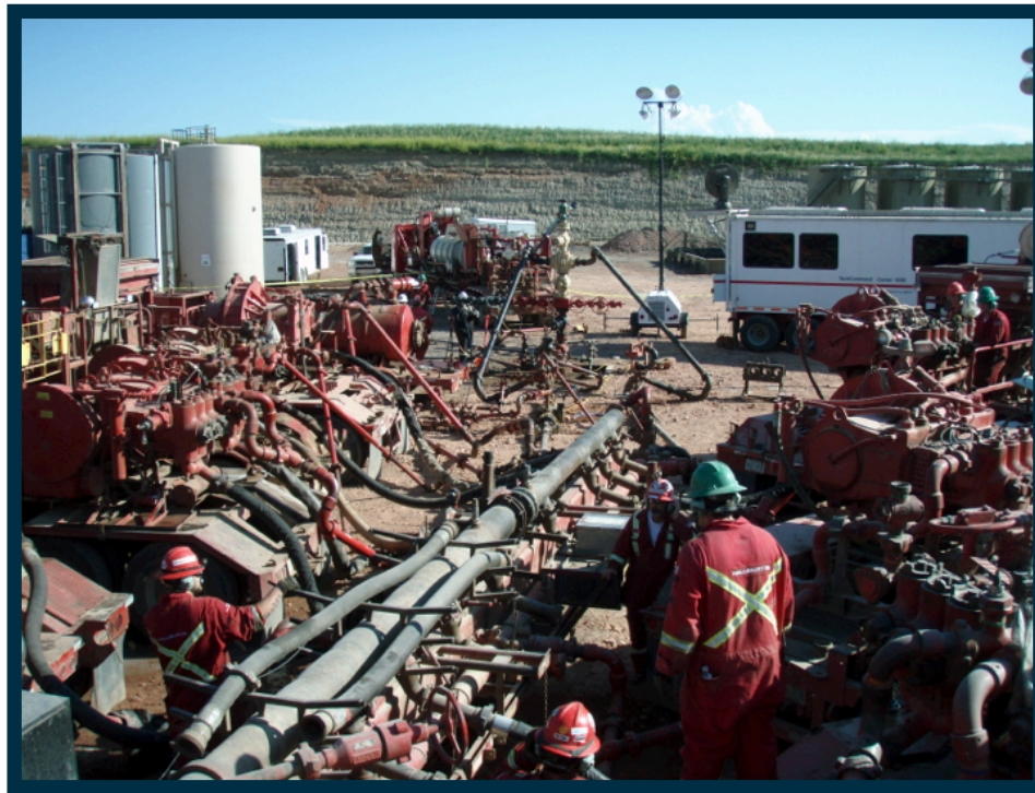
Figure 1-9: Fracturing trucks working together to inject well 5
